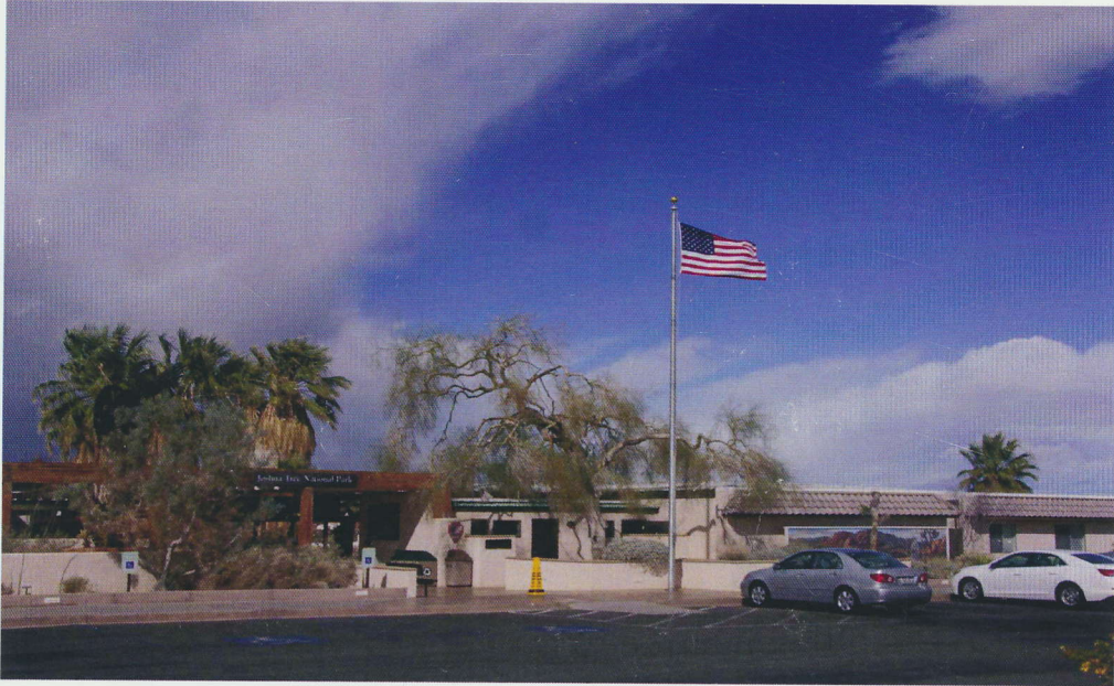
Oasis of Mara administration & visitor center building complex. Twentynine Palms, California. NPS photo. 2014.
