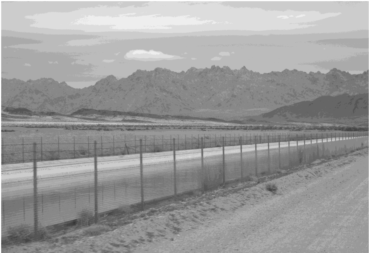
Figure1-11. The Colorado River Aqueduct near the Coxcomb Mountains. The 242-mile project began in 1932 and took seven years to complete. Photo by the author.
