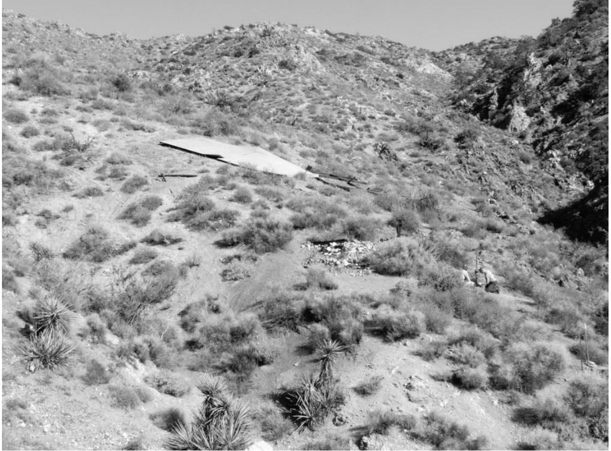
Figure 6-4. A guzzler consists of a broad rock face or piece of sheet metal that directs precipitation or piped water to a tank or trough. Downhill from the metal sheet two Park Service employees conduct repairs. Photographer unknown. JTNP Natural Resource Division files.
