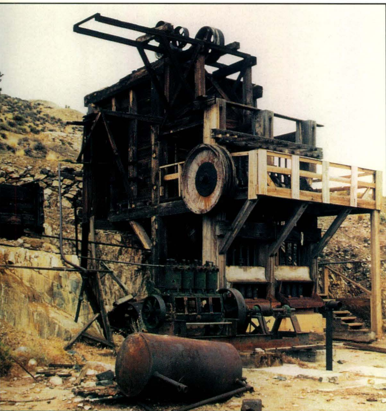
The remains of the Lost Horse Mine and the restored ore bin and 10-stamp mill. Photo by D.D. Trent.
